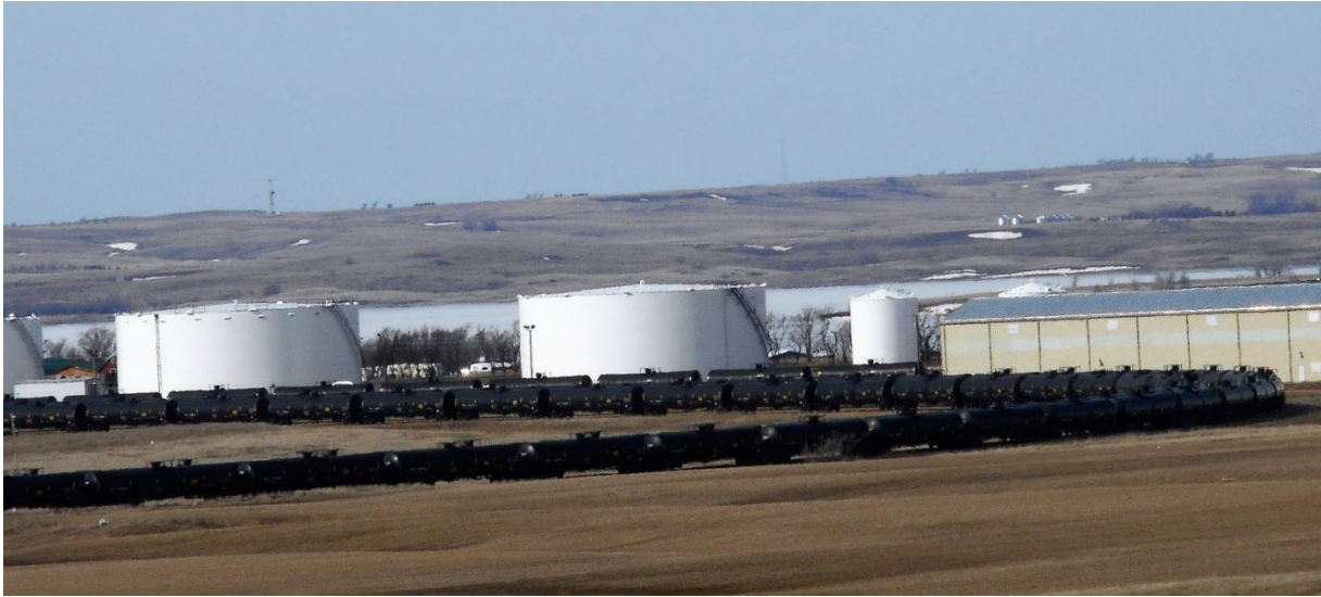
Large storage tanks and rail cars at loading facility near a body of water. Midwest Consortium photo taken from public road in New Town, ND. March 2017.
